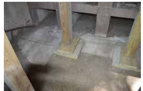
Above: SCAD students taking measurements at the mausoleum. Below: The Library had wooden posts installed to reinforce the roof.
